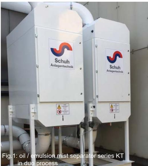
Fig.1: oil / emulsion mist separator series KT in duo process
