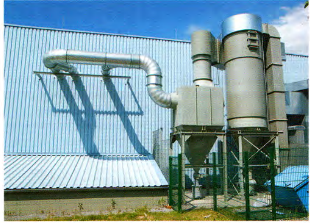
Figure 3. Spark separator and pulse-jet filter
