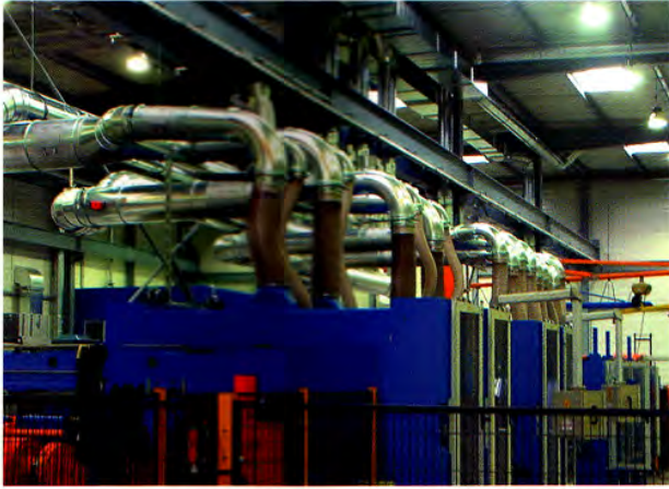
Figure 2. View of the suction device on the production unit
